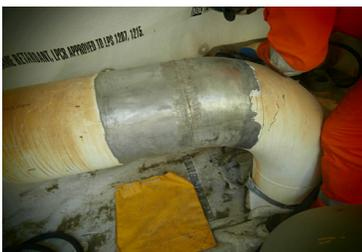
***A qualified ClockSpring|NRI technician applies a proprietary engineered composite repair system on a damaged line offshore***
