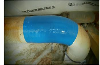
**A completed composite repair on a corroded line offshore restores line integrity**
