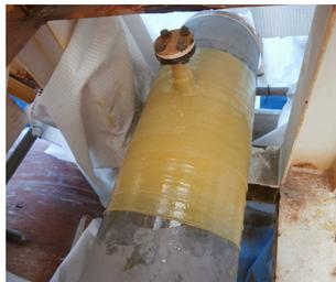
**Composite repairs are specifically designed for complex geometries and can be installed effectively on lines where other repair methods are impractical or**
