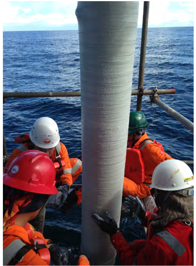
Figure 3. The polyurethane system within the A+ Wrap system utilises moisture to start the polymerisation reaction and can function in wet environments.
