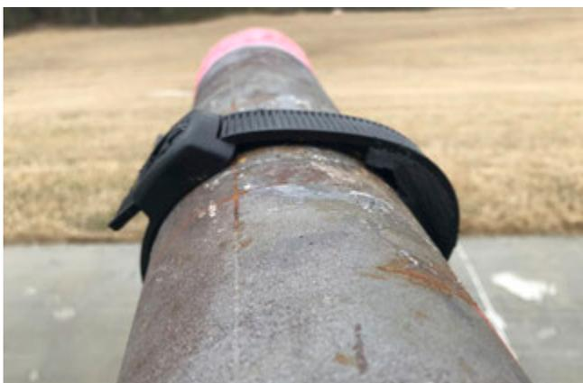
Figure 3. A completed Leak Stopper installation has a low profile that allows it to be overwrapped with a composite for a long-lasting repair.
