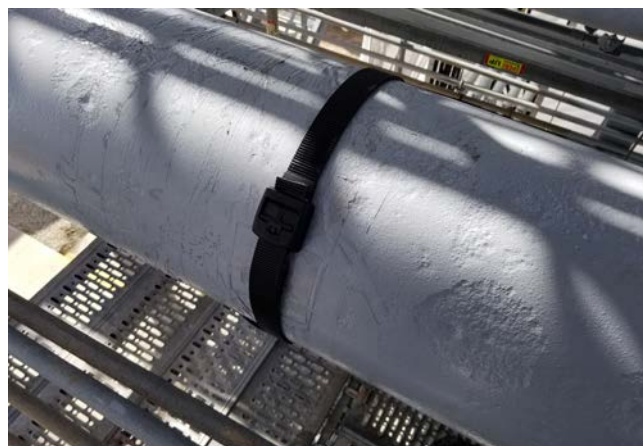
Figure 4. A repair in the field awaits a composite overlay.
