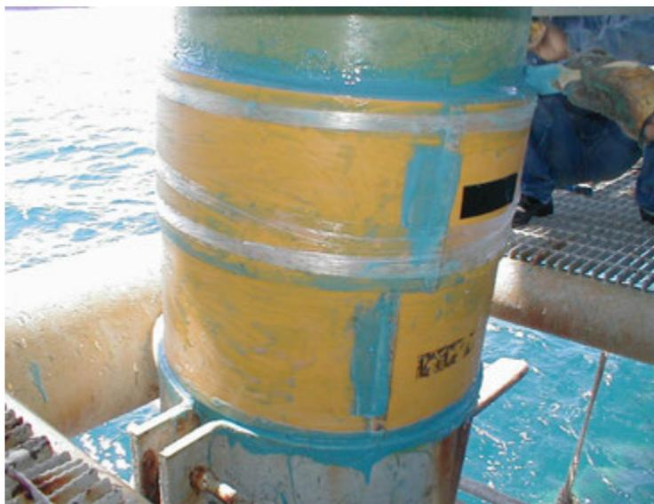
**Figure 5.** Clock Spring composite repair sleeves arrive on site ready to install, eliminating heavy lifting and welding risks and delivering a completed repair in a matter of hours. Photo courtesy of Clock Spring Company, Inc.
