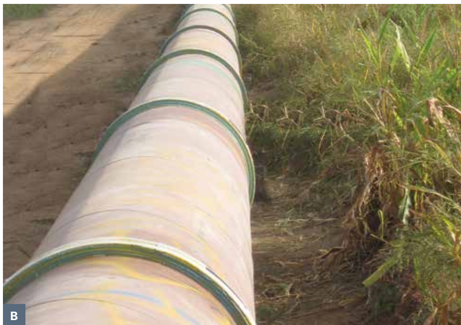
A: Workers installing the Clock Spring spacer system.
