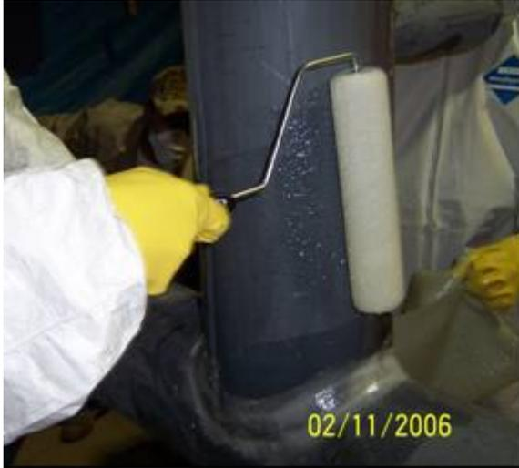
Figure 18. Apply a layer of resin to pipe surface first
