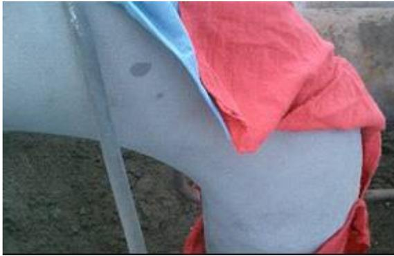
Figure 3. Pipe after grit blasting. Note water drip on pipe required surface to be re-blasted before repair application
