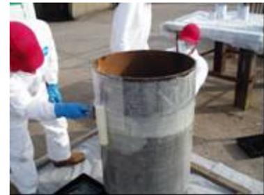
Figure 10. Apply more resin to fabric and work in
