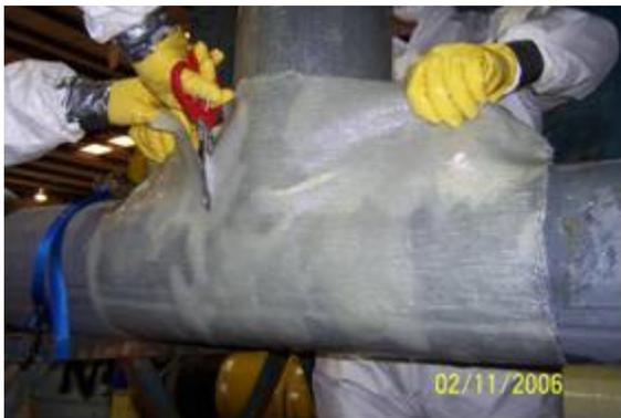
Figure 39. Build up layers alternating between trunk and branch.
