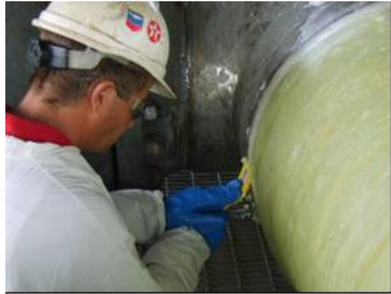
Figure 4. Fairing – thickened resin being applied around weld beads.
