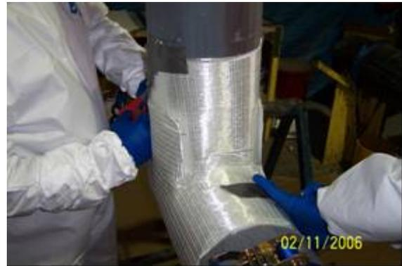
Figure 38. Apply fabric to trunk and slit to form overlap onto branch.
