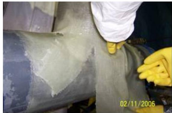
Figure 40. Build up layers alternating between trunk and branch (remember to allow for tapers on both).
