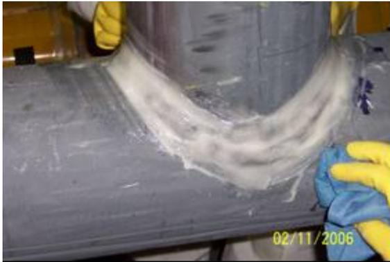
Figure 35. Fair connection to 5mm radius minimum.
