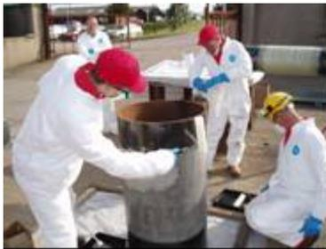
Figure 8. Apply layer of resin to pipe
