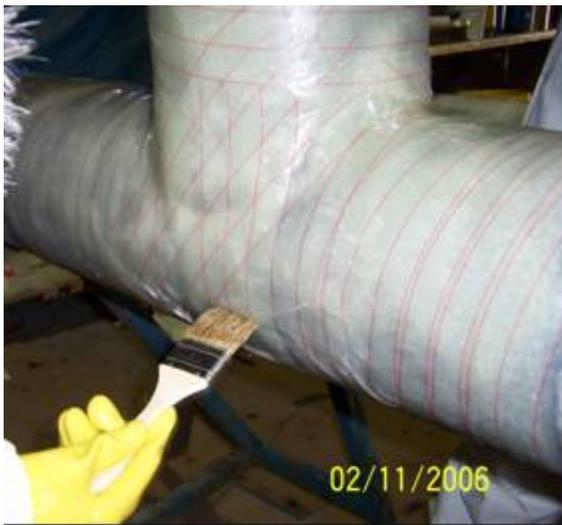
Figure 43. Ensure surface is fully 'wet' with resin and peel ply is flat over all surfaces.
