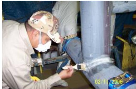
Figure 14. Filler smoothed using a paint brush
