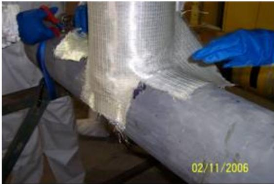
Figure 37. Cut fabric so that tabs of material extend onto trunk.
