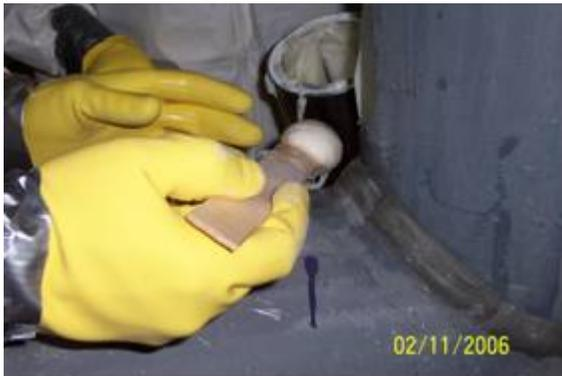
Figure 13.. Filler applied to fair in uneven edge
