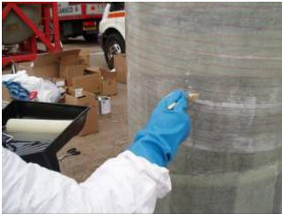
Figure 23. Apply more resin where required
