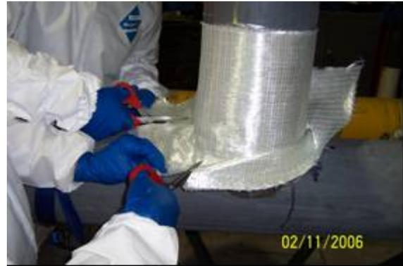
Figure 36. Wrap fabric around branch and slit fabric back to connection so that it lays flat on the surface.
