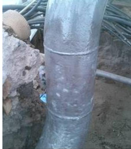
Figure 19. Pipe with resin applied prior to application of glass
