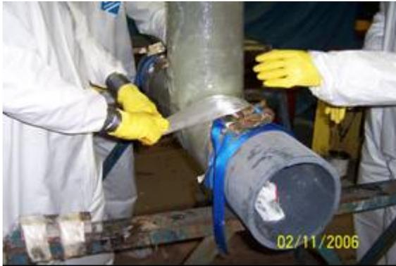
Figure 41. Apply peel ply.
