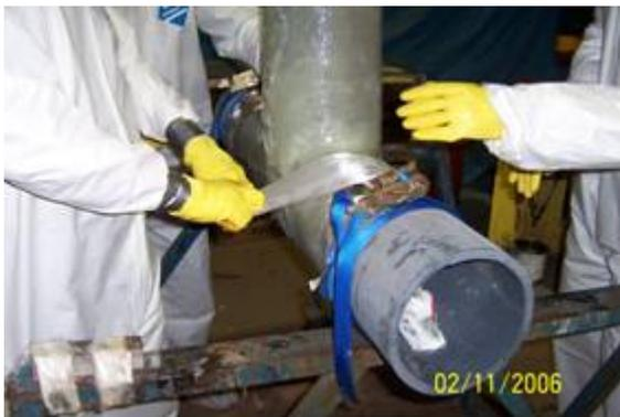
Figure 25. Using peel ply to consolidate fabric in tee
