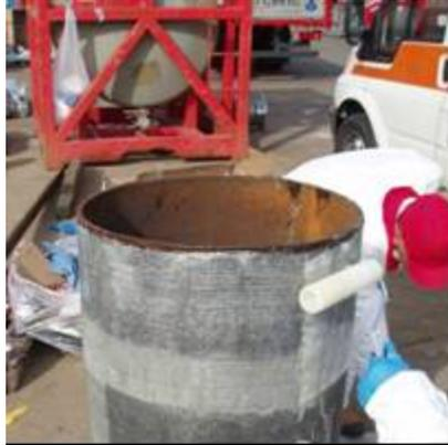
Figure 15. Consolidation using a roller
