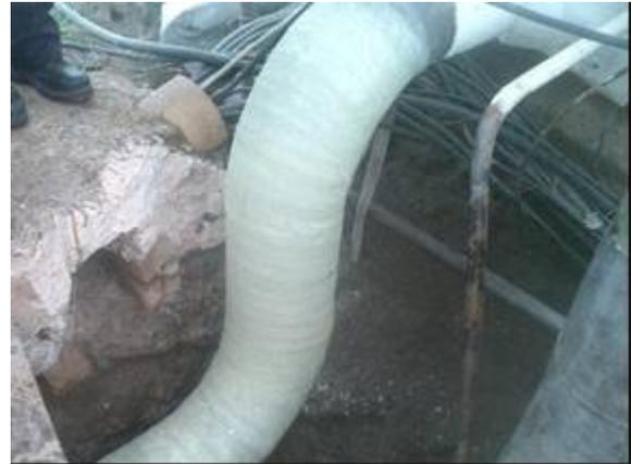
Figure 31. Completed spiral wrap repair
