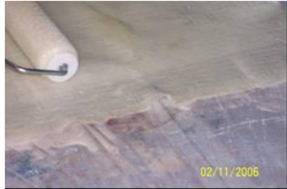
Figure 7. Resin wets out cloth when pressure applied with roller
