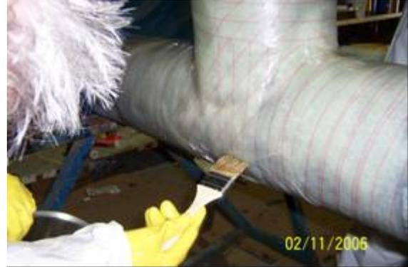
Figure 16. Consolidation using a paint brush
