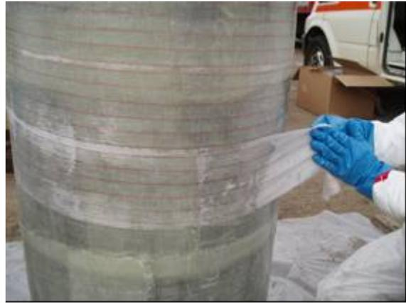
Figure 22. Application of peel ply. Resin can be seen to be coming through fabric
