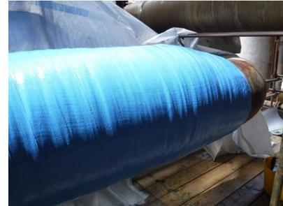
ClockSpring|NRI technicians applied UV stable epoxy coating to add further protection to repair.
