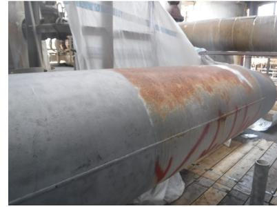
Technicians carefully grit blast the line as close as possible to the defect without creating further damage or causing production loss on the damaged line.
