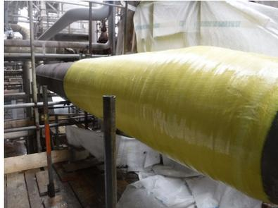
The completed installation restored a length of 3.1 m (10.2 ft) 711-mm of corroded (28-inch) carbon steel line to safe service.
