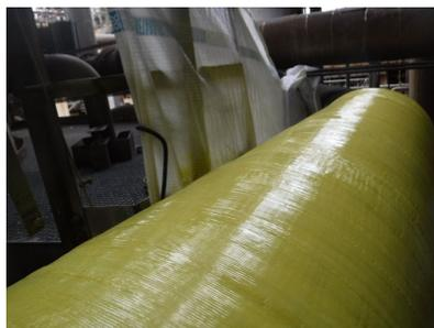
Technicians installed a 40-layer system of Thermo-Wrap Inspectable over 3.1 m (10.2 ft) of the damaged line.
