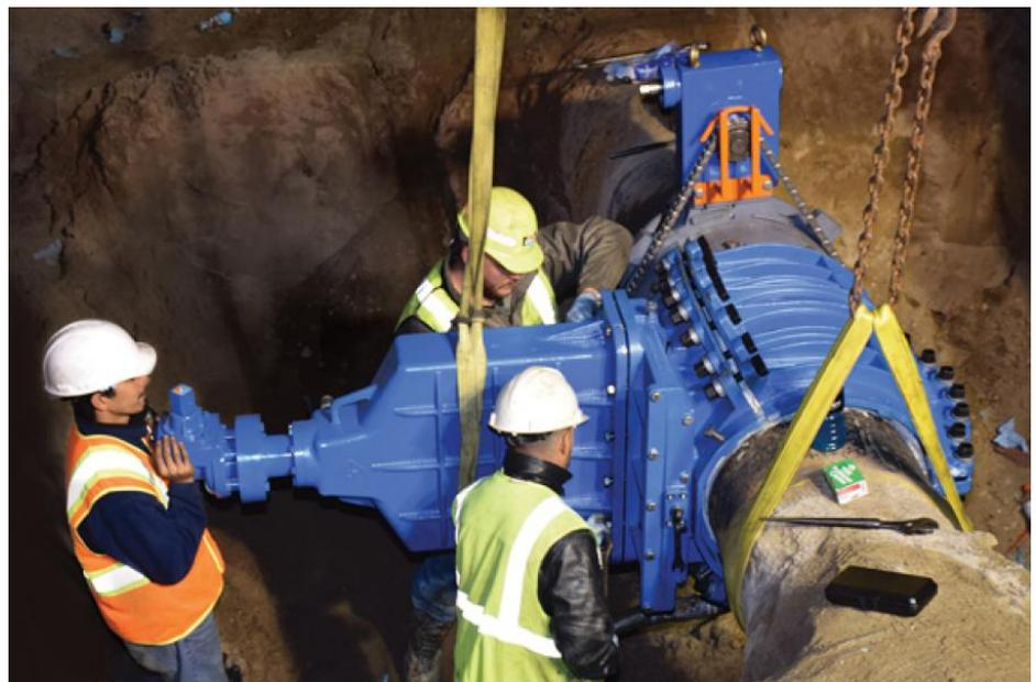
A modification allowed the EZ Valve™ to be installed horizontally on the trunk line.
