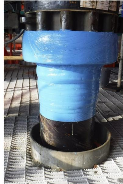
In the final step of the 355-mm (14-inch) line repair, technicians applied 2 layers of UV stable epoxy to protect the repair from future corrosion and abrasion.
