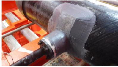
Technicians used a proprietary injection leak arrest system to seal the live leaks and Syntho-Poxy™ 101 to improve the complex geometry of the lines.
