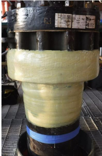
With the leak sealed, technicians applied 8 layers of Thermo-Wrap™ Inspectable ECR to the 355-mm (14-inch) line.
