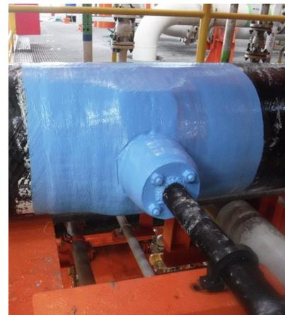
With the Thermo-Wrap™ Inspectable ECR installed on the joint between the 508-mm (20-inch) and 51-mm (2-inch) GRE lines, technicians covered the repair with 2 layers of UV-stable epoxy to protect the repair from future corrosion and abrasion.
