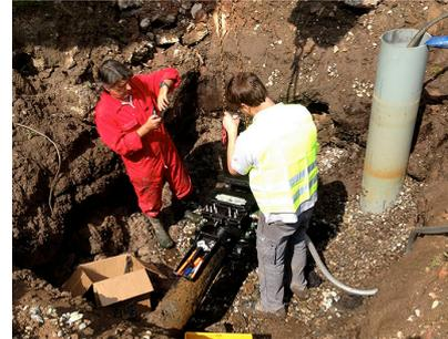
Wedge gate is lowered and drip tight seal is created.
