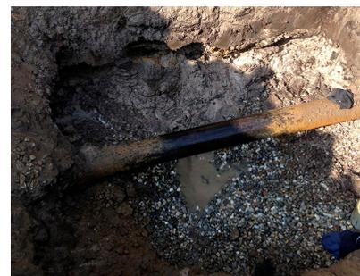
Excess Water is drained, pipe is thoroughly cleaned and prepped for valve body.
