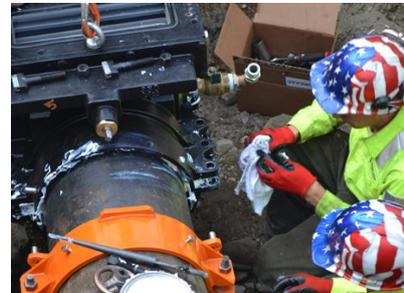
The installation team places the valve body to begin the installation on the 100-year-old cast iron pipe.
