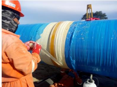
Clock Spring-trained and certified technicians from local distributor, Nirsa, apply spacers to a pipeline covered with Contour WA™.
