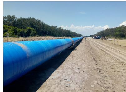
A 500-m (1,641-foot) section of 1,067-mm (42-inch) diameter gas pipeline coated with Contour WA to protect the fusion bonded epoxy (FBE) coat. The blue film is installed over the wrap while curing.
