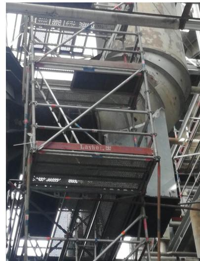
Because of the location of the line, special scaffolding was built to give technicians access so they could wrap 508-mm (20-inch) wide swathes of fiber carbon cloth around the 2,000-mm (78.7-inch) diameter flare line.
