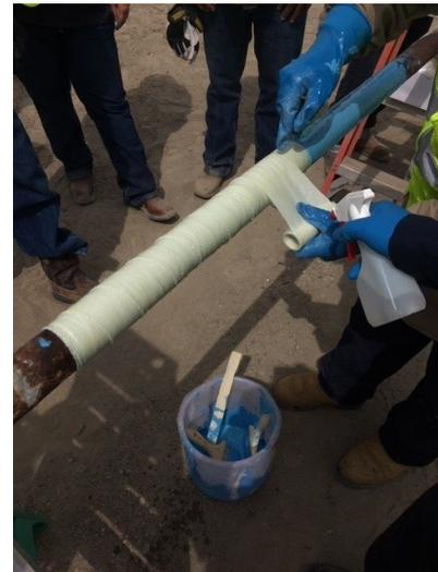
Clock Spring trained and certified technician apply Contour WA™ to a prepared line.
