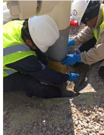
Installers secure Snap Wrap to strengthen the pipe and protect it at the air/soil interface.
