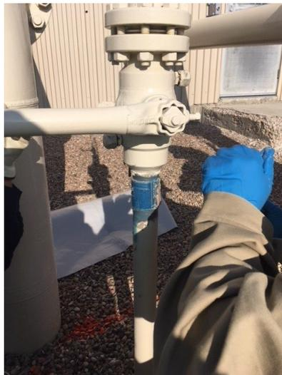
Pipe supports are installed to limit the effects of corrosion and the environment for the gas transmission lines.
