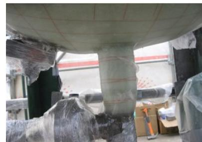
The damaged area was wrapped with the Contour wet applied repair system, with technicians applying filler material over the corroded section, followed by quad-axial stitched fiberglass cloth affixed with a two-part epoxy.
