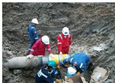
Certified installers place bridge units on each side of the weld.
