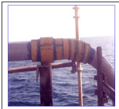
Figures 1a, b, c Bend Repairs
