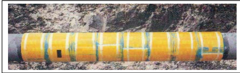
Figure 1. Multiple Clock Spring® Units
