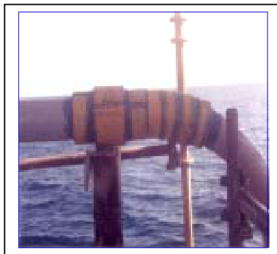
Figures 1a, b, c Bend Repairs
