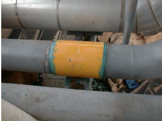
8 inch Snap Wrap Repair
