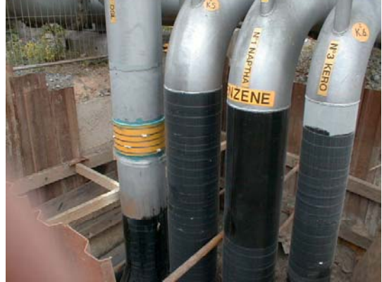
18 inch Snap Wrap Repair
