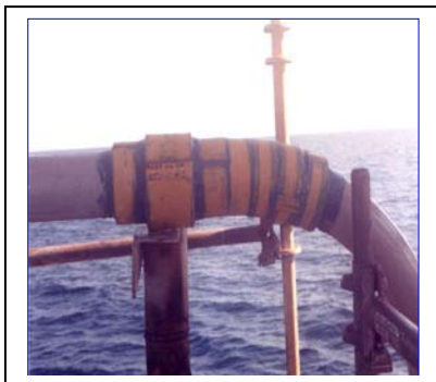
Figures 2a, 2b. Reinforcement of Bends
