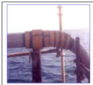
Figures 1a, b, c Bend Repairs
